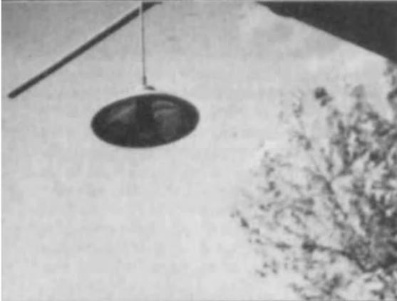
Plate 24. Electric bowl heater photographed by day with current on. Reflections on the underside are not caused by the heated element. (b)
