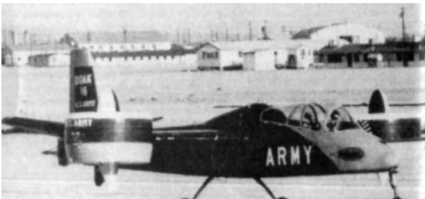
Plate 4. VTOL sequence of the experimental DOAK aircraft with ducted swivel rotors.
