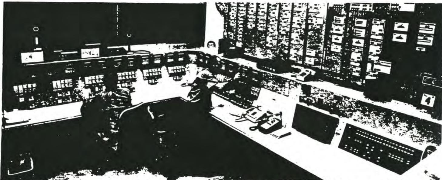
Nerve center: This computer control board, designed especially for Disney World, keeps tabs on the entire \$20-million power system. Other computers monitor the park's rides, run a fire-prevention system that is tied into a private fire department as large as Orlando's, and run the Disney World laundr
