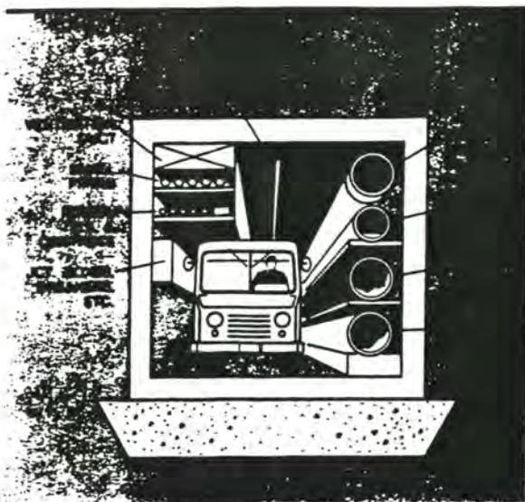
Cross-section of underground utilidor shows separate storm sewage. Clean water from roofs and amusement rides runs into Bay Lake. Oily runoff water from parking lots goes into holding ponds for treatment.
