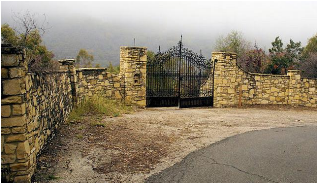
Security gates still stand at the former entrance to the compound.
