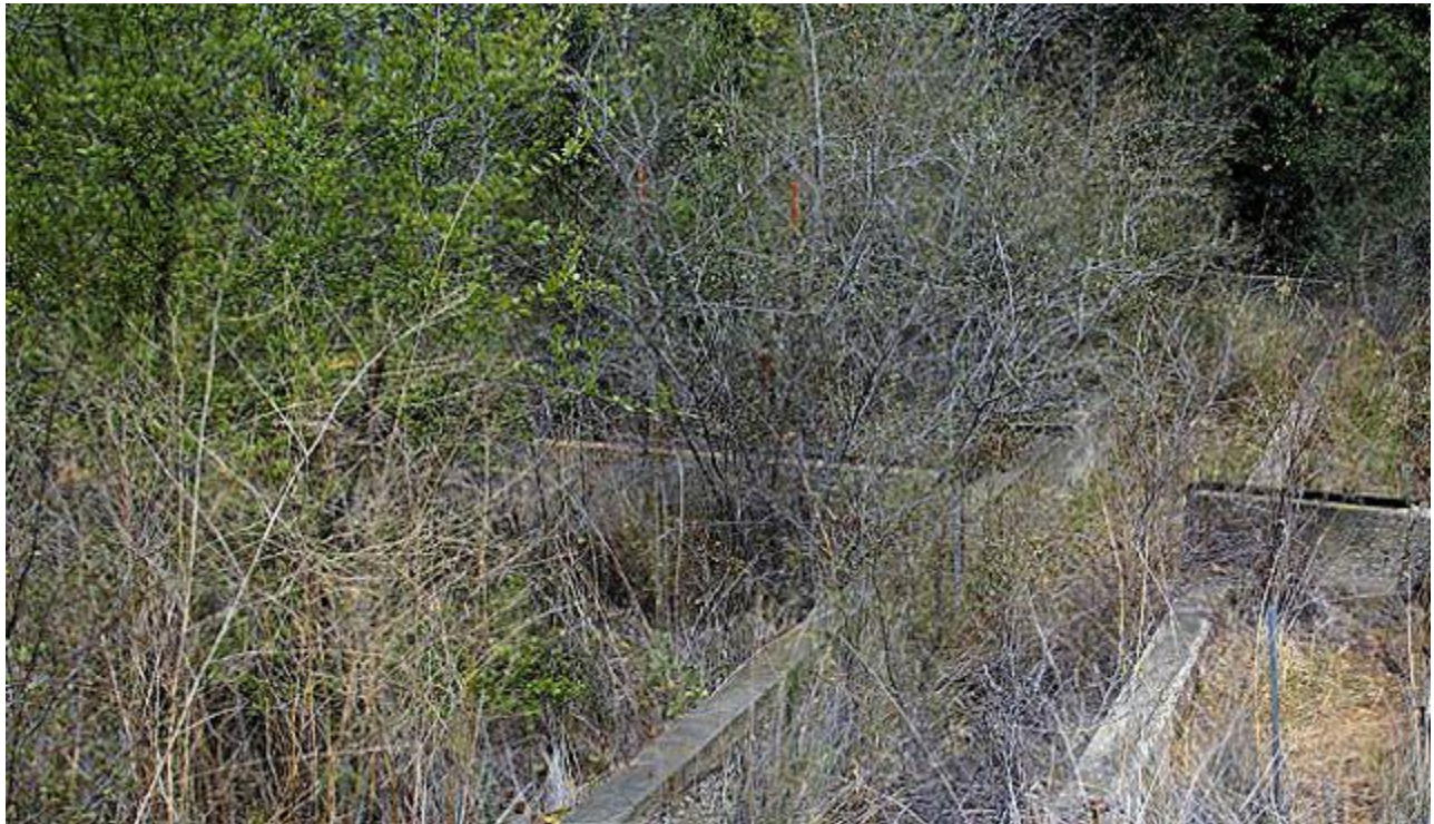
A portion of the over-grown foundation of what was once a state-of-the-art greenhouse.
