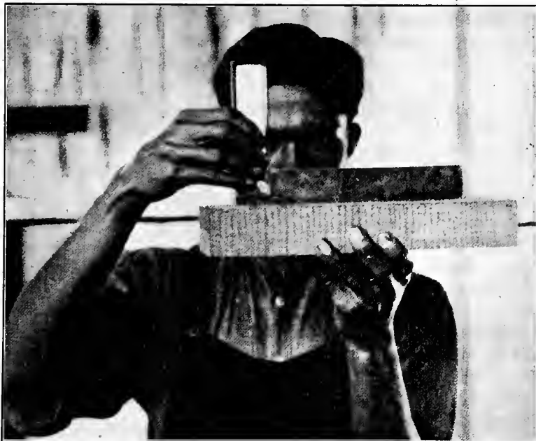
Fig. 110. Testing for straightness.
