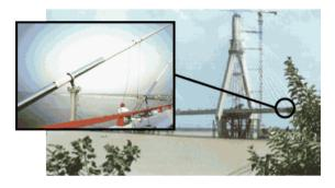
Fig. 7: The Dongting Bridge with MR Dampers.
