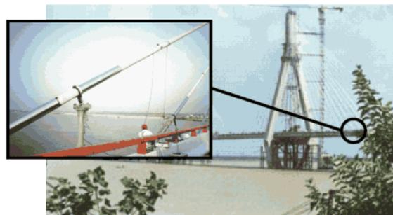
**Fig. 7:** The Dongting Bridge with MR Dampers.
