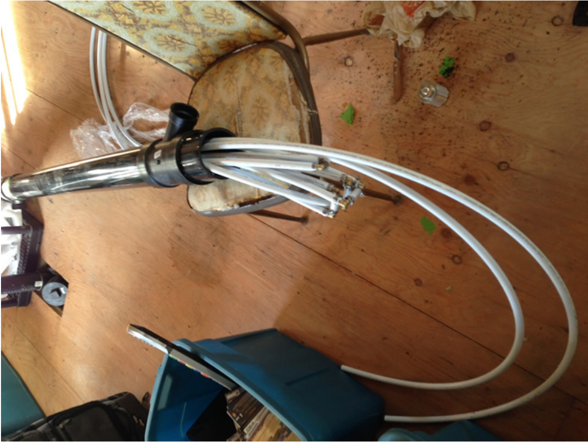
The bundle of PEX being placed in the new shower drain. Once the bundle is in place, a cap with holes for the two PEX lines is installed and sealed with silicone caulk.
