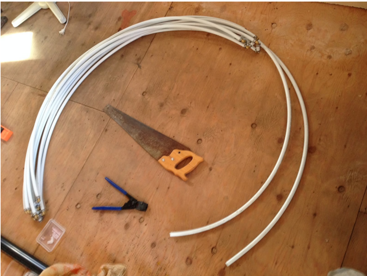
Putting together the bunndle of PEX that will be placed in the new section of shower drain. The PEX connected with brass fittings with crimp rings.
