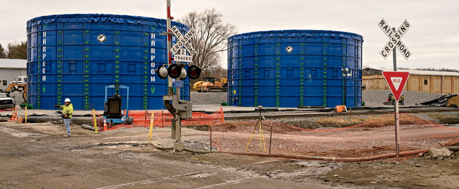
Two blue tanks temporarily hold wastewater collected from the cleanup site that has yet to be treated or sent for disposal.
