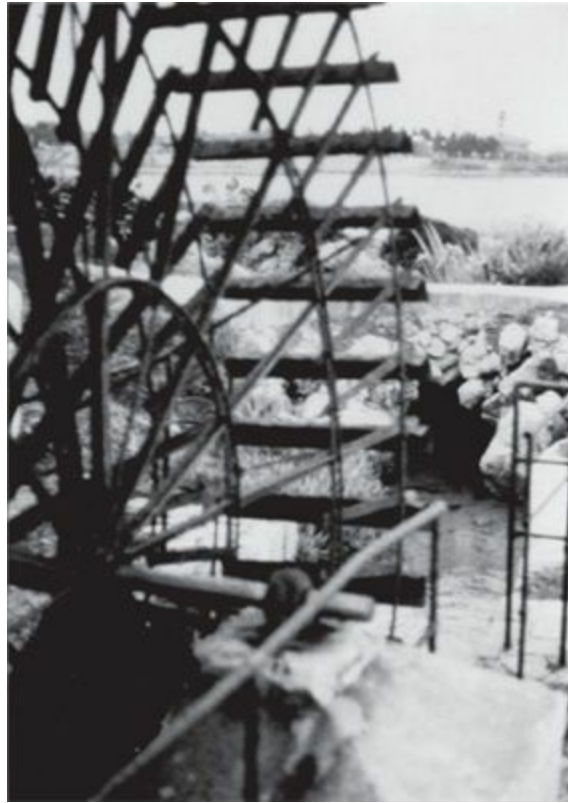
Figure 1.10. Waterwheel on Cephallonia Island built over a sluiceway to generate electricity from inflowing water. The water level drops about 2 meters below sea level by the time it reaches the waterwheel and thereafter drops several more meters before entering a fissure. (Photo by the author)
