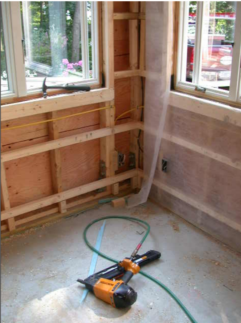
the insul-mesh is stapled and pulled tight..
