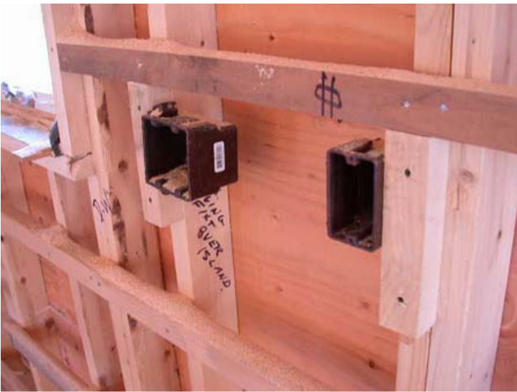
the electrician roughs in , the boxes can be mounted on 2x2 blocking...
