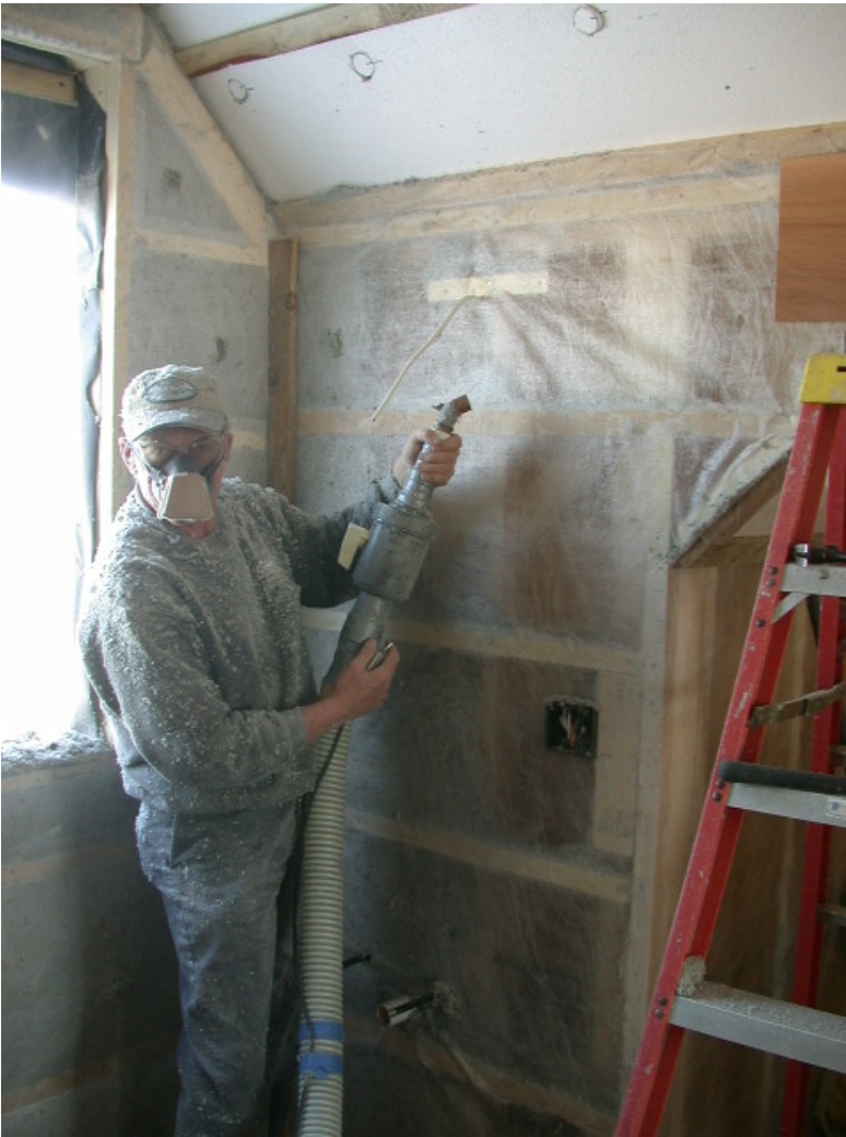
We use one hole every 16" ...and work one stud bay at a time.. going from filled to empty
