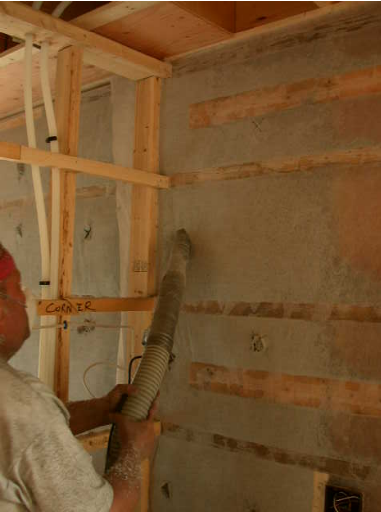
and topping out...
