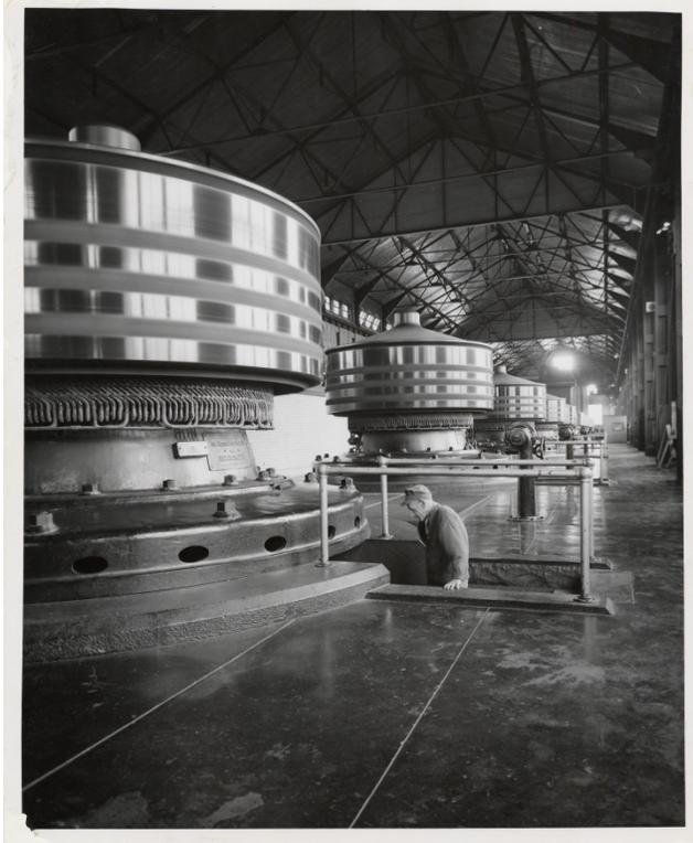
**Figure 3** Westinghouse/Tesla generators at Niagara Falls
